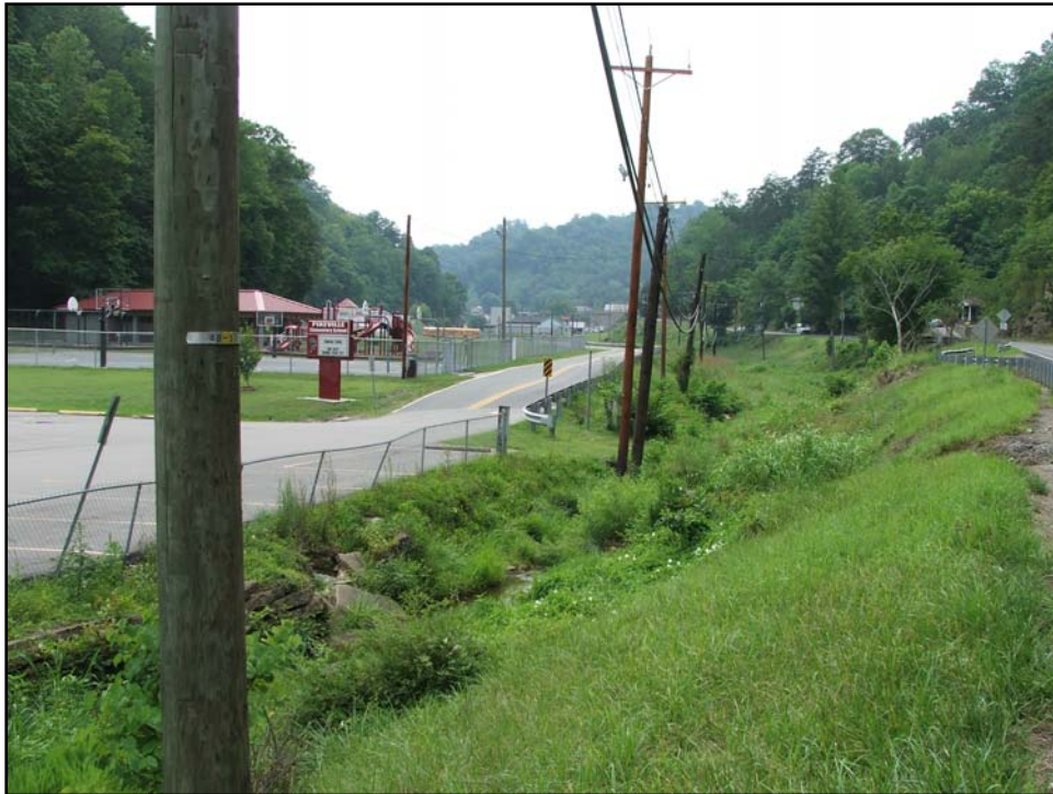
View West along KY 1460 and Chloe Creek
