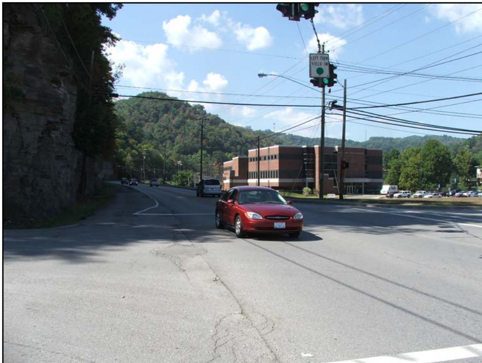
Southern KY 1426 approach at Huffman Avenue/Summit Drive intersection
