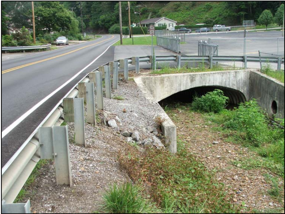
Chloe Creek Culvert, passing under KY 1460.
