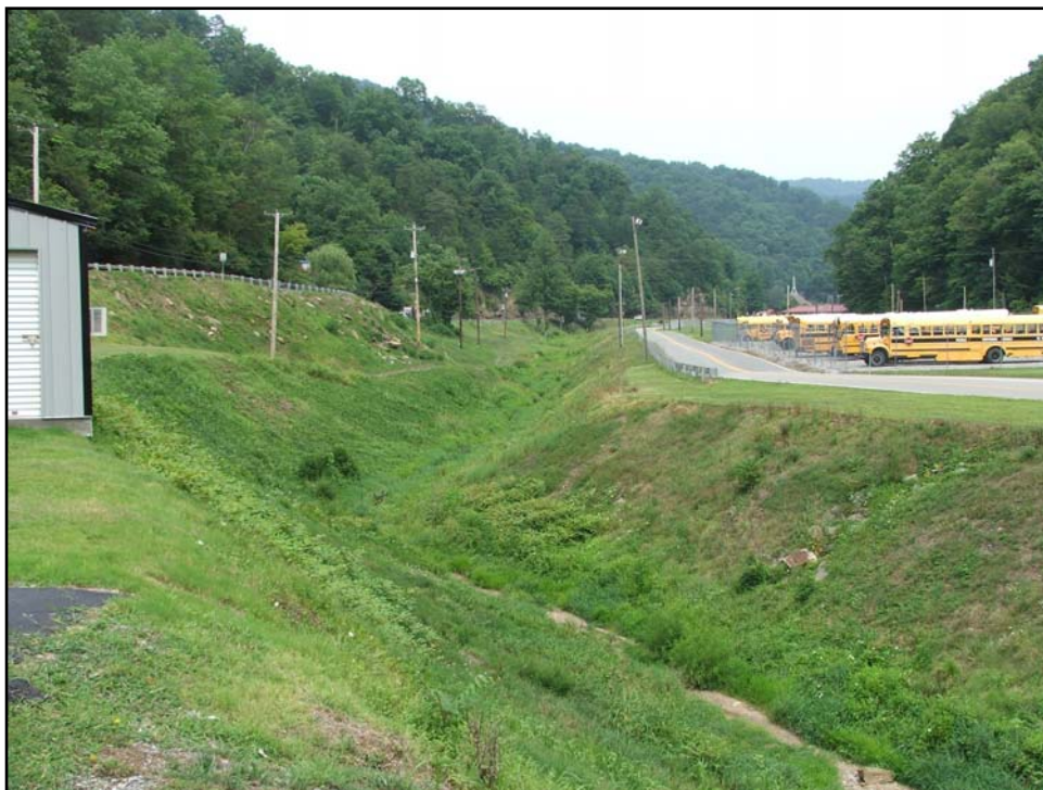
Area between KY 1460 and school access road facing east
